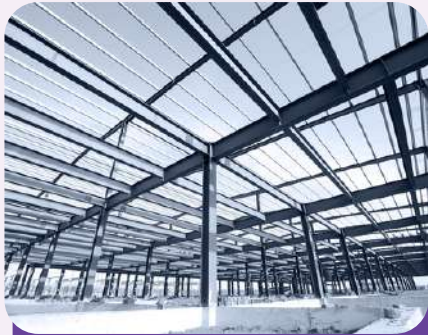
Any type of Steel Structures
