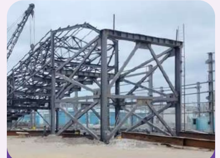
Pipe rack / Conveyor Structures
