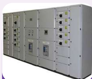
SwitchGear Cabinet Components
